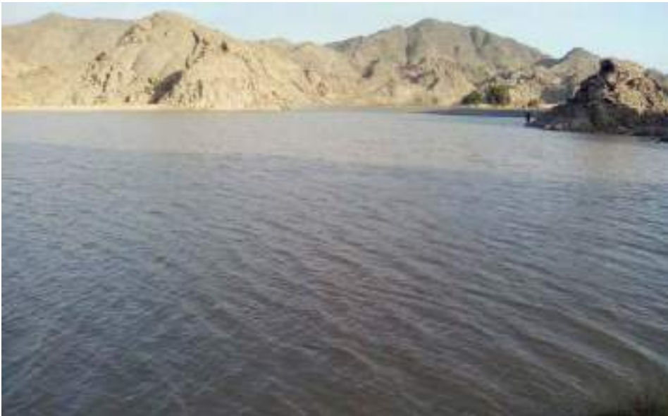
Water reservoir constructed in Chagai, Balochistan under Drought Resilience Agricultural Modeling DRAM Project.
